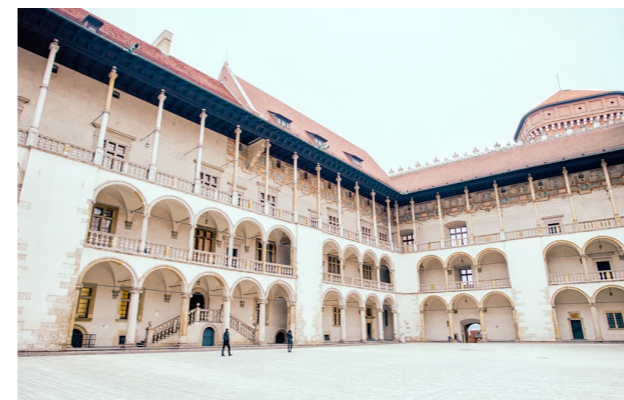
The colonnade on the courtyard of Wawel castle.
